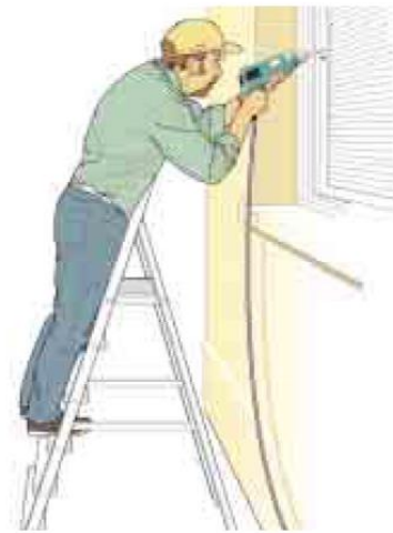
Figure 2b Correct - steps facing work activity
